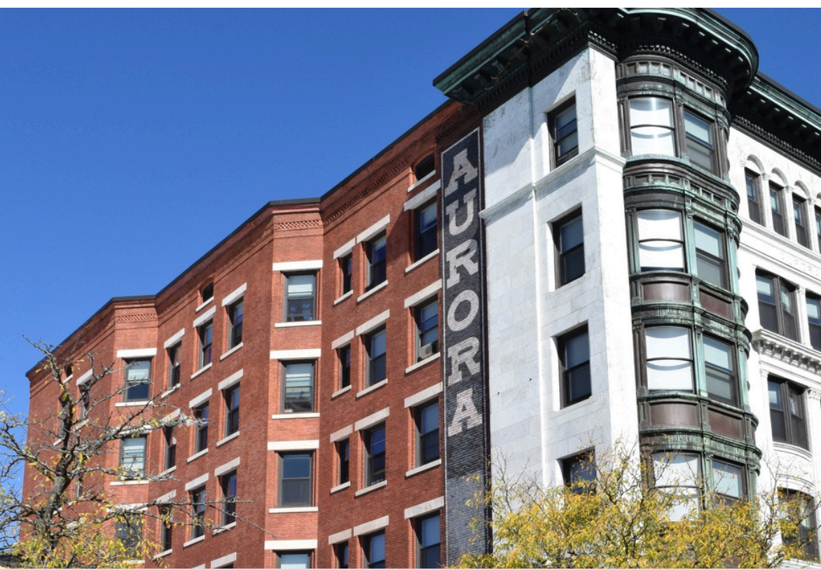
THE AURORA APARTMENTS, WORCESTER, MA
