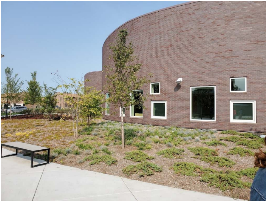
Windows are complete. Sidewalks and landscaping are in place.
