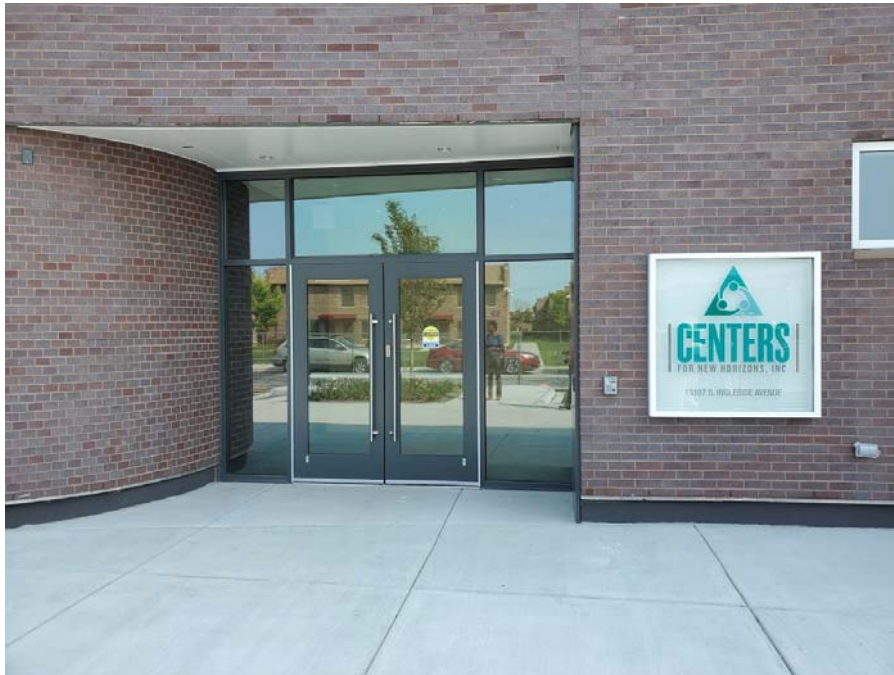
Entrance systems and signage are complete.
